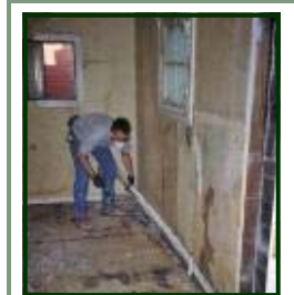
For large areas, consult with remediation professionals.
